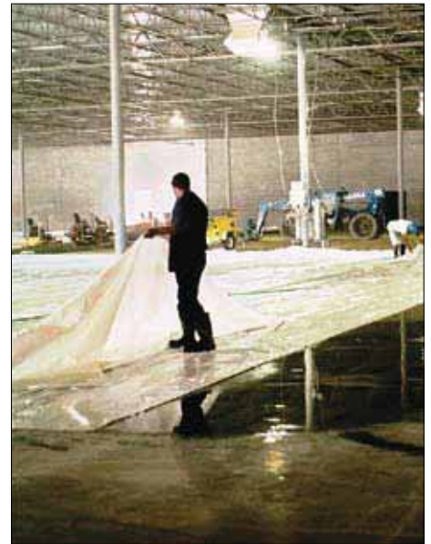
Apply pre-wetted curing covers polyethylene side up.
