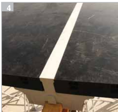
4 Block the panels onto the Y-beams
