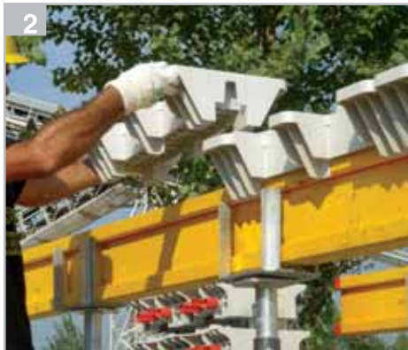
2 Place the H-beam
