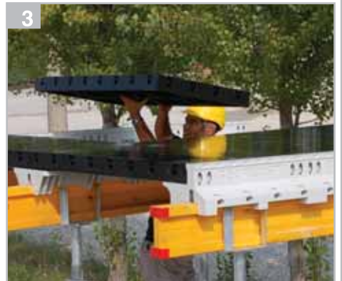
3 Place the GEOPANEL® 120 panel
