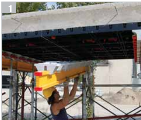
1 Remove the H-beams
