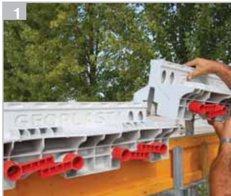
1 Place pre-assembled Y-beam and wedges
