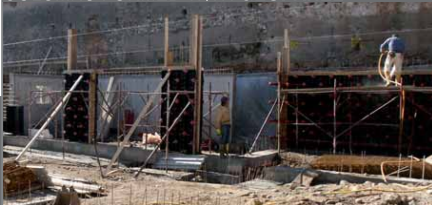
COLUMNS FORMED WITH GEOPANEL®
